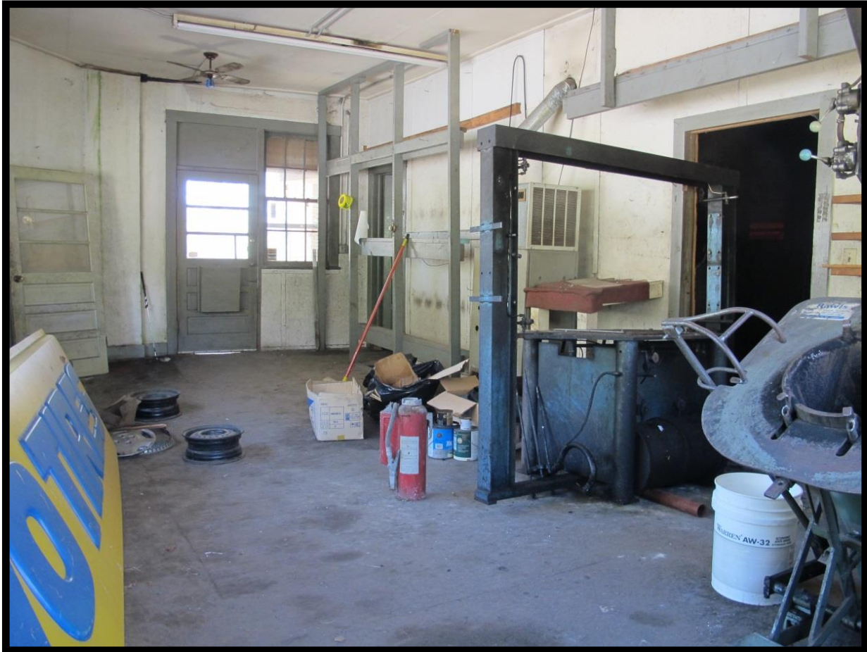
Figure 24: Bobby Burns Filling Station, Interior of Larger Wing.
