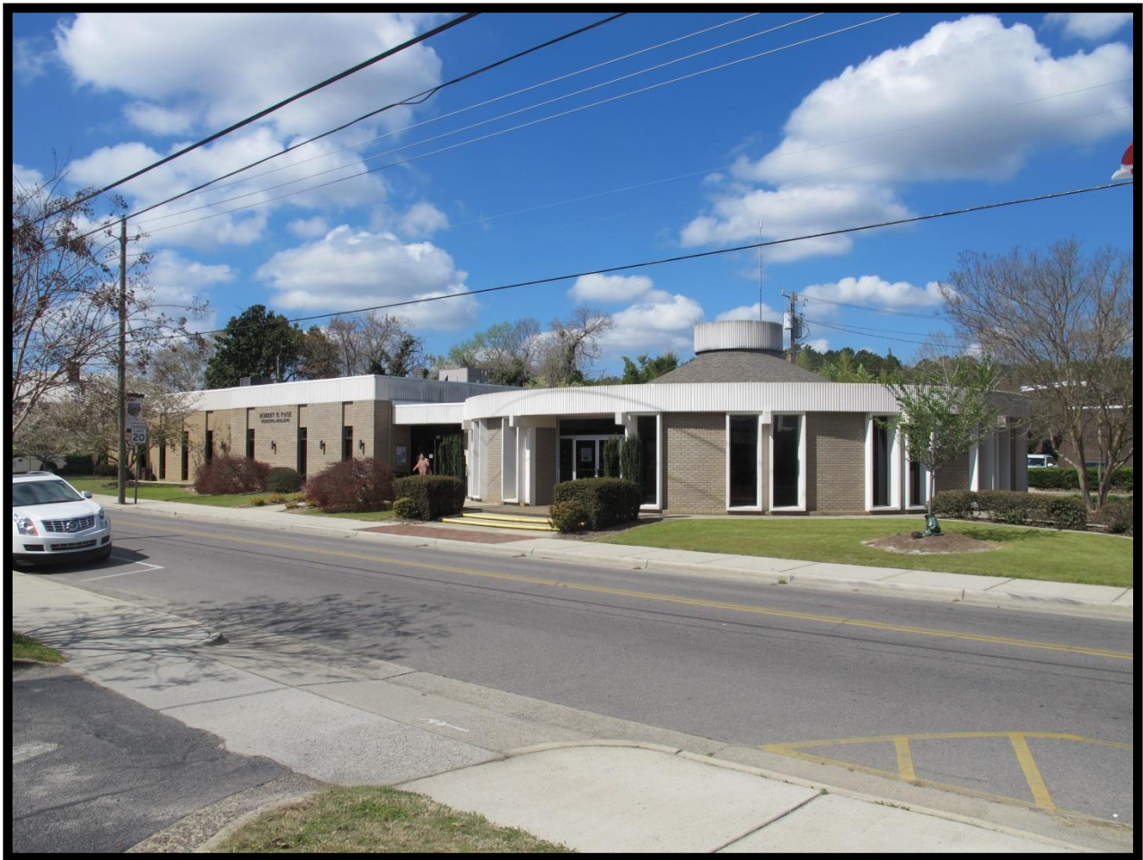
Figure 46: Former Citizens Bank & Trust Company of Southern Pines, Looking Southwest.
