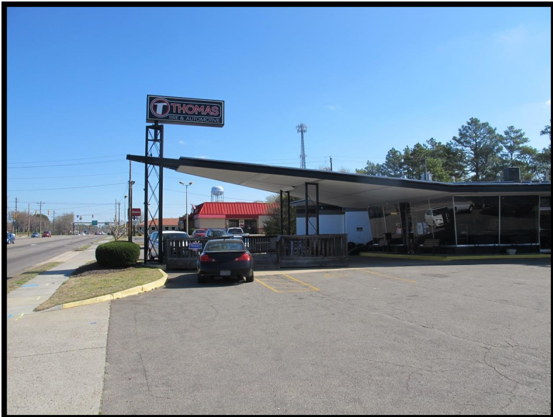
Figure 8: Phillips 66 Service Station, View of Canopy Looking Northeast.
