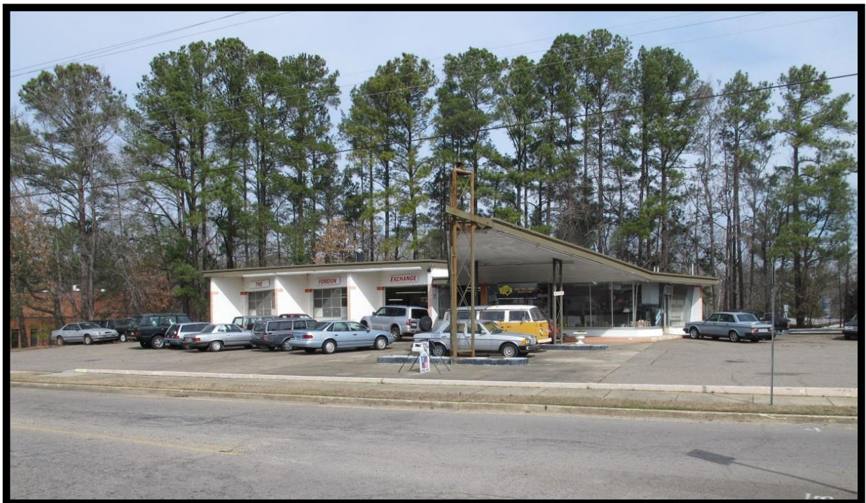
Figure 14: View of a (former) Phillips 66 Service Station at the Corner of Carbondon Street and Carthage Street in Sanford, Lee County, North Carolina.
