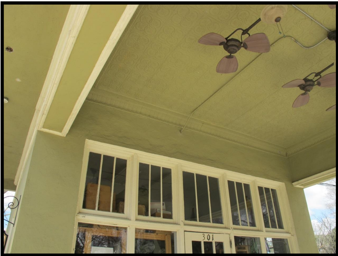
Figure 33: Poplar Street Service Station (MR0123), View of Pressed-Tin Ceiling.
