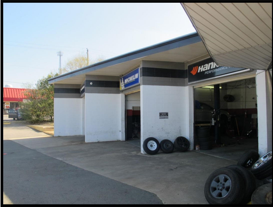
Figure 5: Phillips 66 Service Station, View of Garage Bays Looking Northeast.
