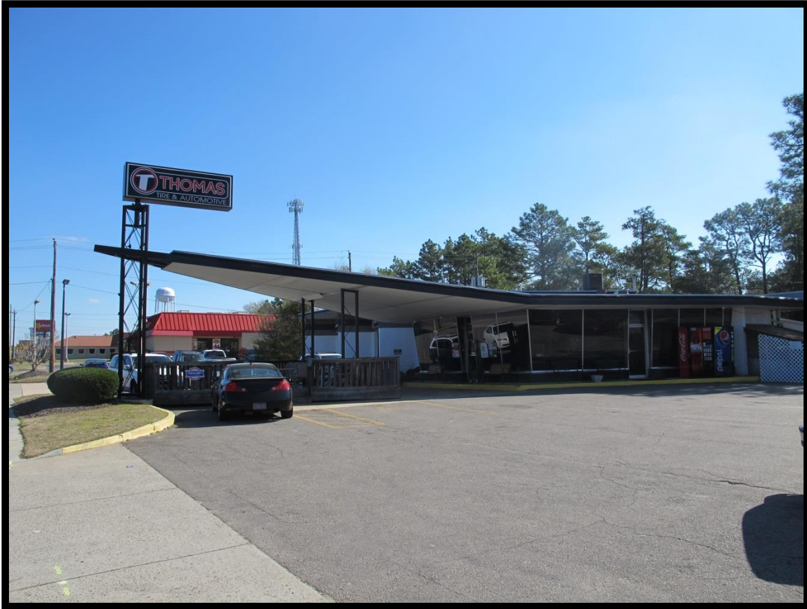
Figure 3: Phillips 66 Service Station, Looking Northeast.
