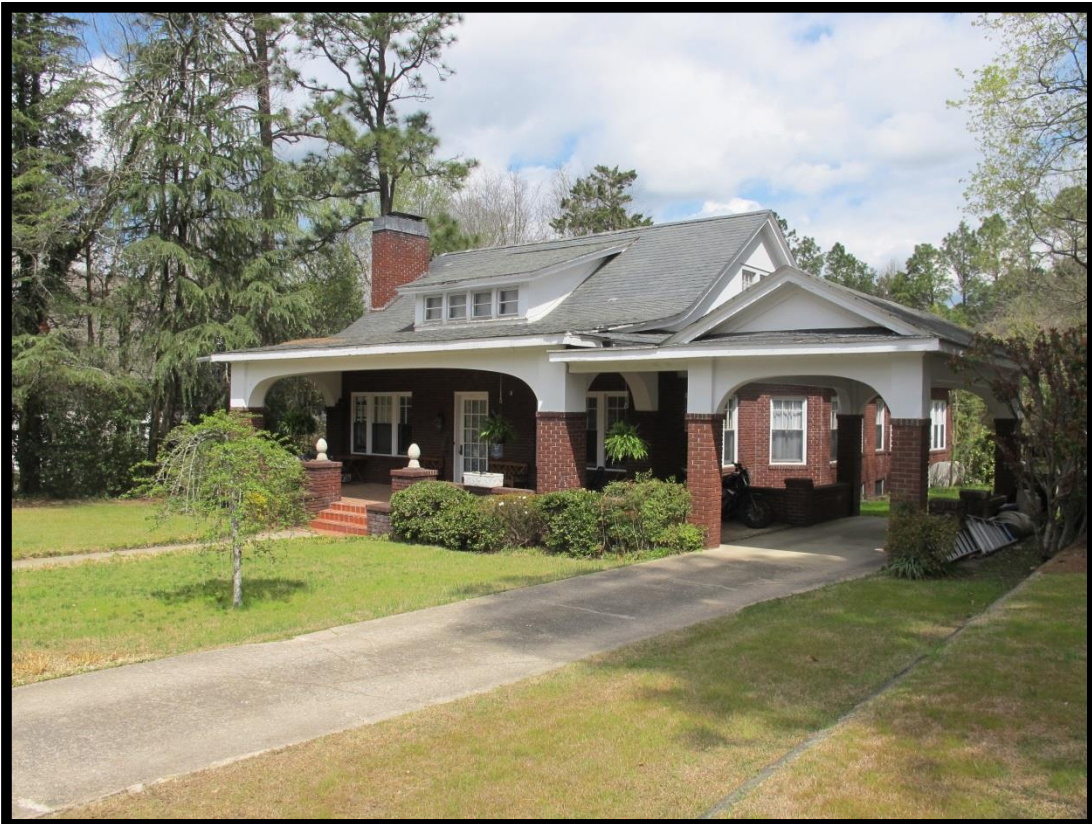
Figure 43: McKeithan-Guion House (MR0084), Looking Northwest.
