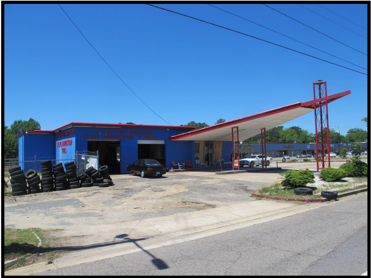
Figure 15: View of a (former) Phillips 66 Service Station at the Corner of Lee Avenue and Judd Street in Sanford, Lee County, North Carolina.
