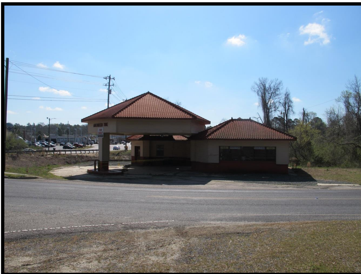
Figure 17: Bobby Burns Filling Station, Looking East.
