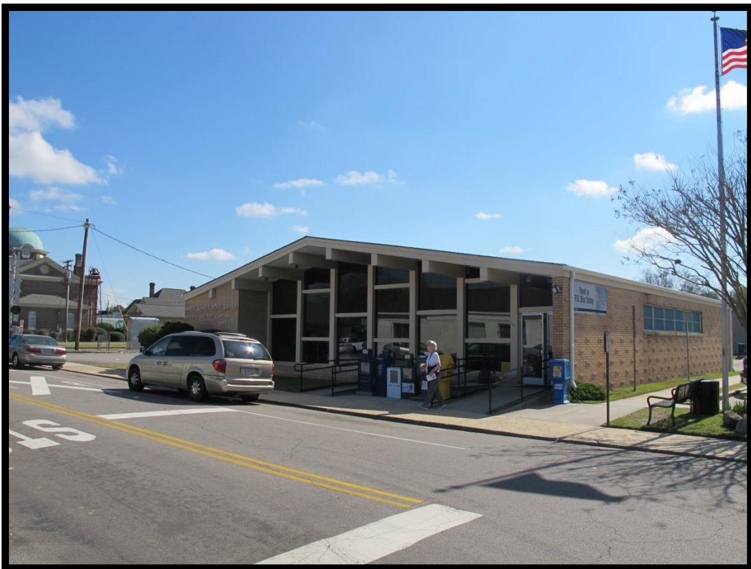
Figure 48: United States Post Office, Looking Northeast.
