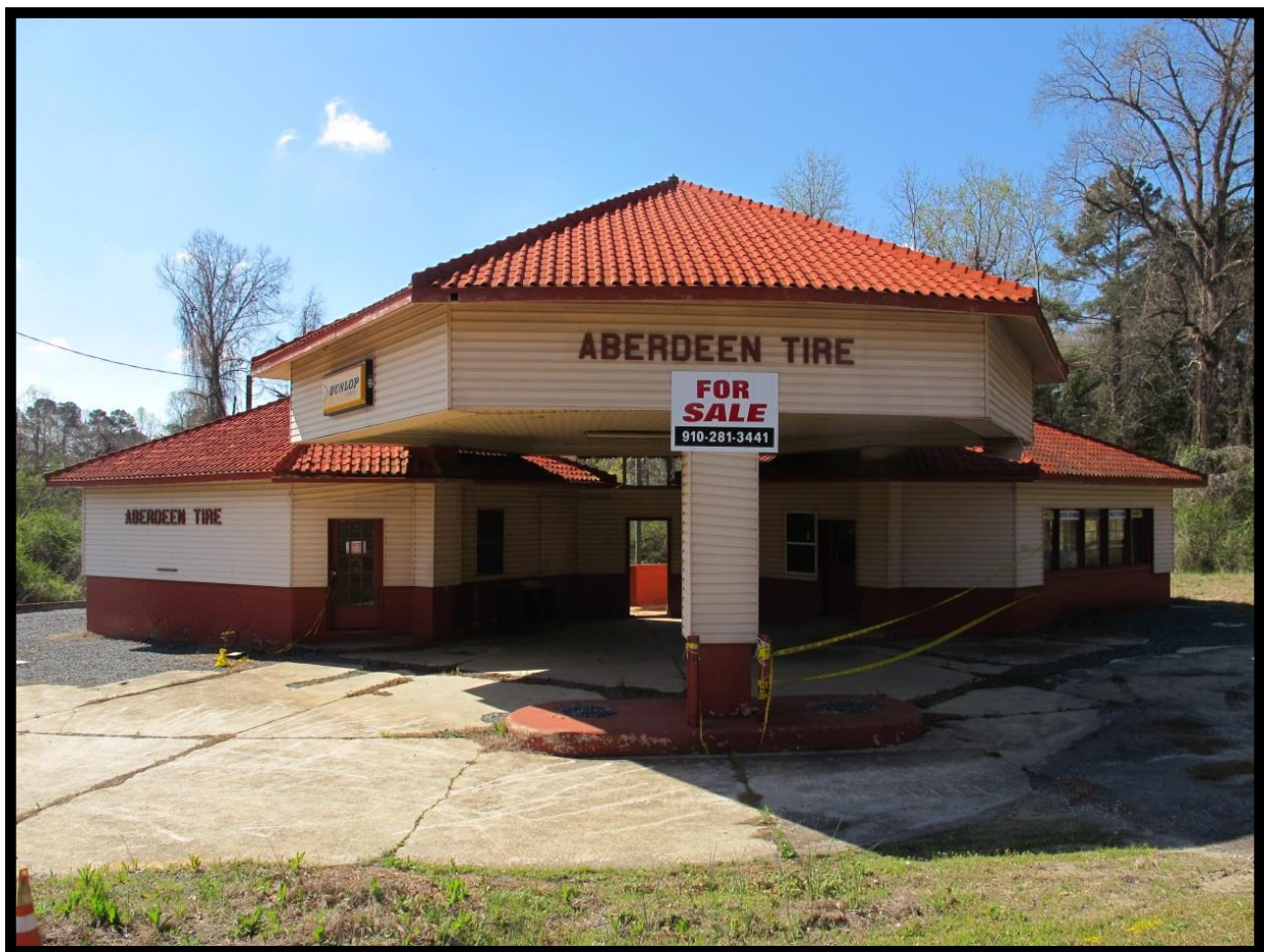
Figure 19: Bobby Burns Filling Station, Looking South.
