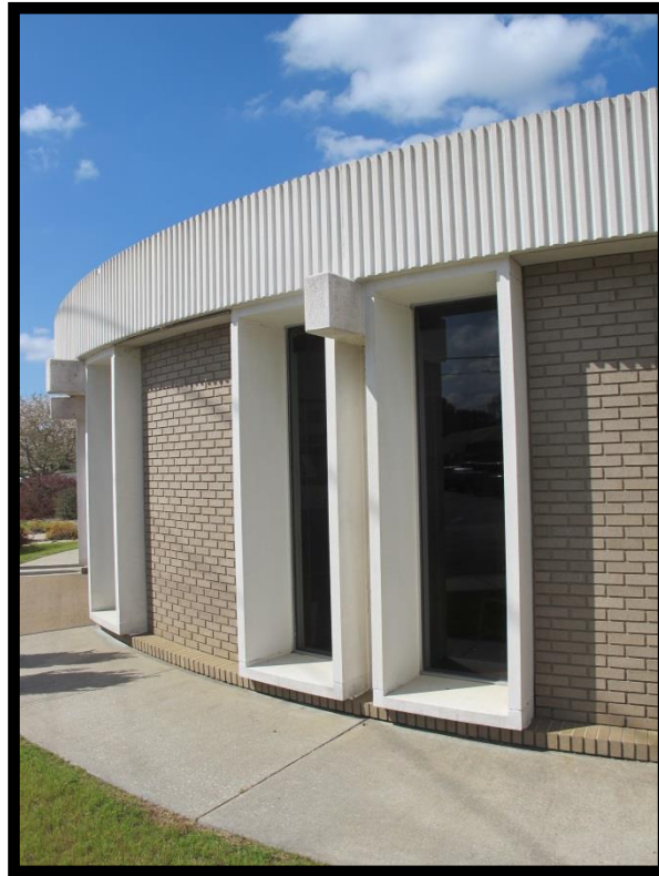
Figure 47: Detail of the Former Citizens Bank & Trust Company of Southern Pines, Looking Southwest.
