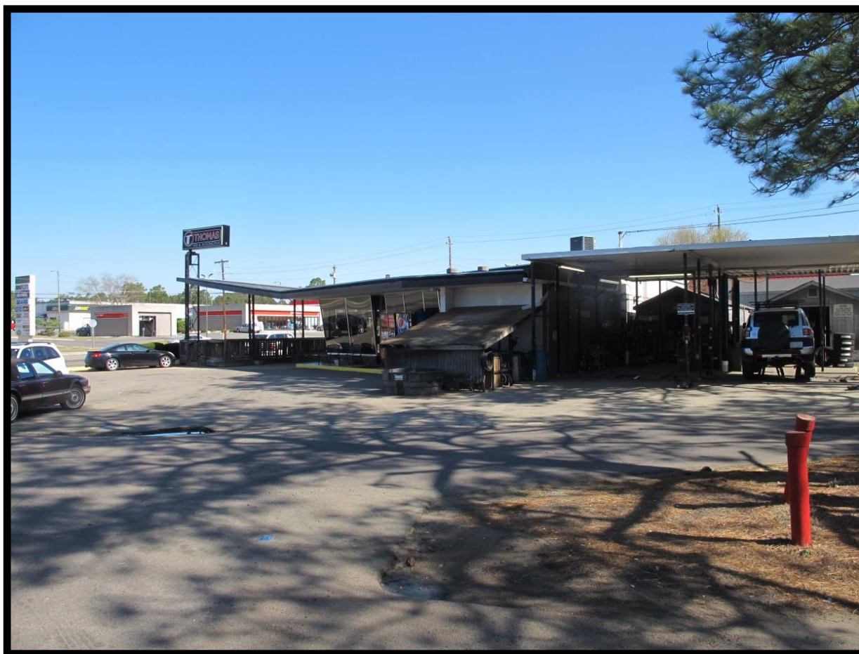
Figure 10: Phillips 66 Service Station, View of Additions and Ancillary Structures Looking Northwest.
