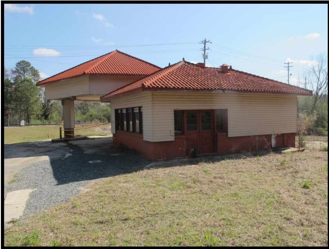
Figure 22: Bobby Burns Filling Station, Looking East.
