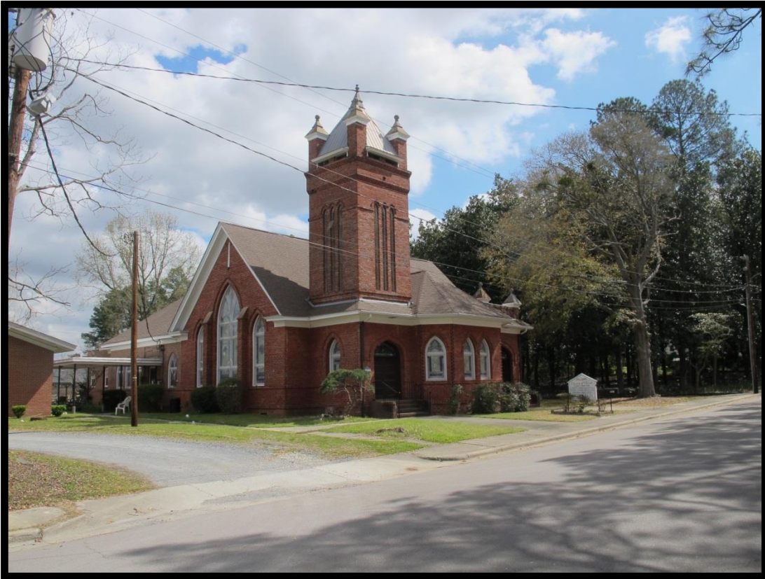
Figure 42: Bethesda Presbyterian Church (MR0074), Looking Northeast.
