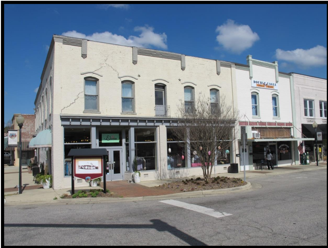
Figure 38: Farrell Building (MR0130), Looking Northwest.
