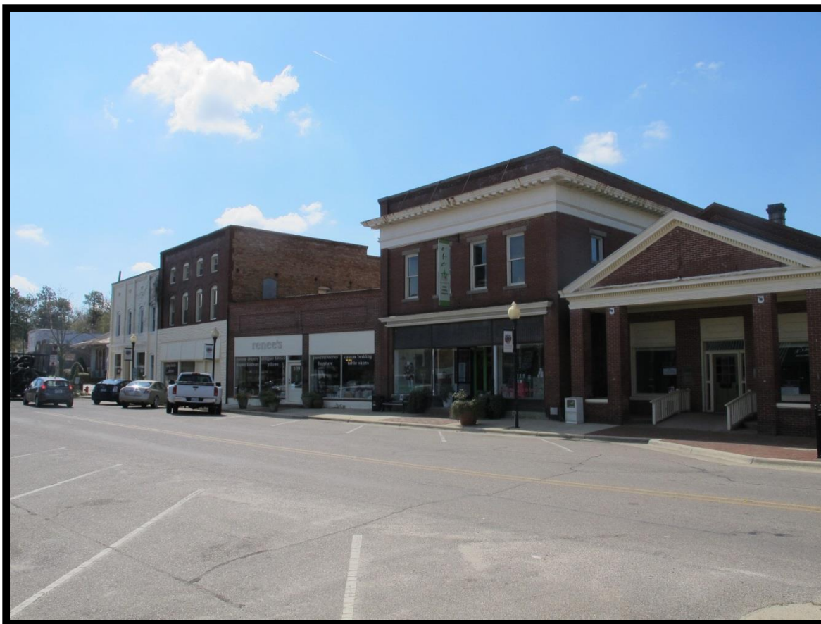
Figure 34: View of Commercial Buildings Along Main Street in the Aberdeen Historic District (MR0141), Looking Southeast.
